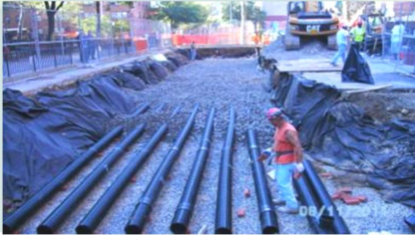
Bronx River Houses perforated pipe systems
