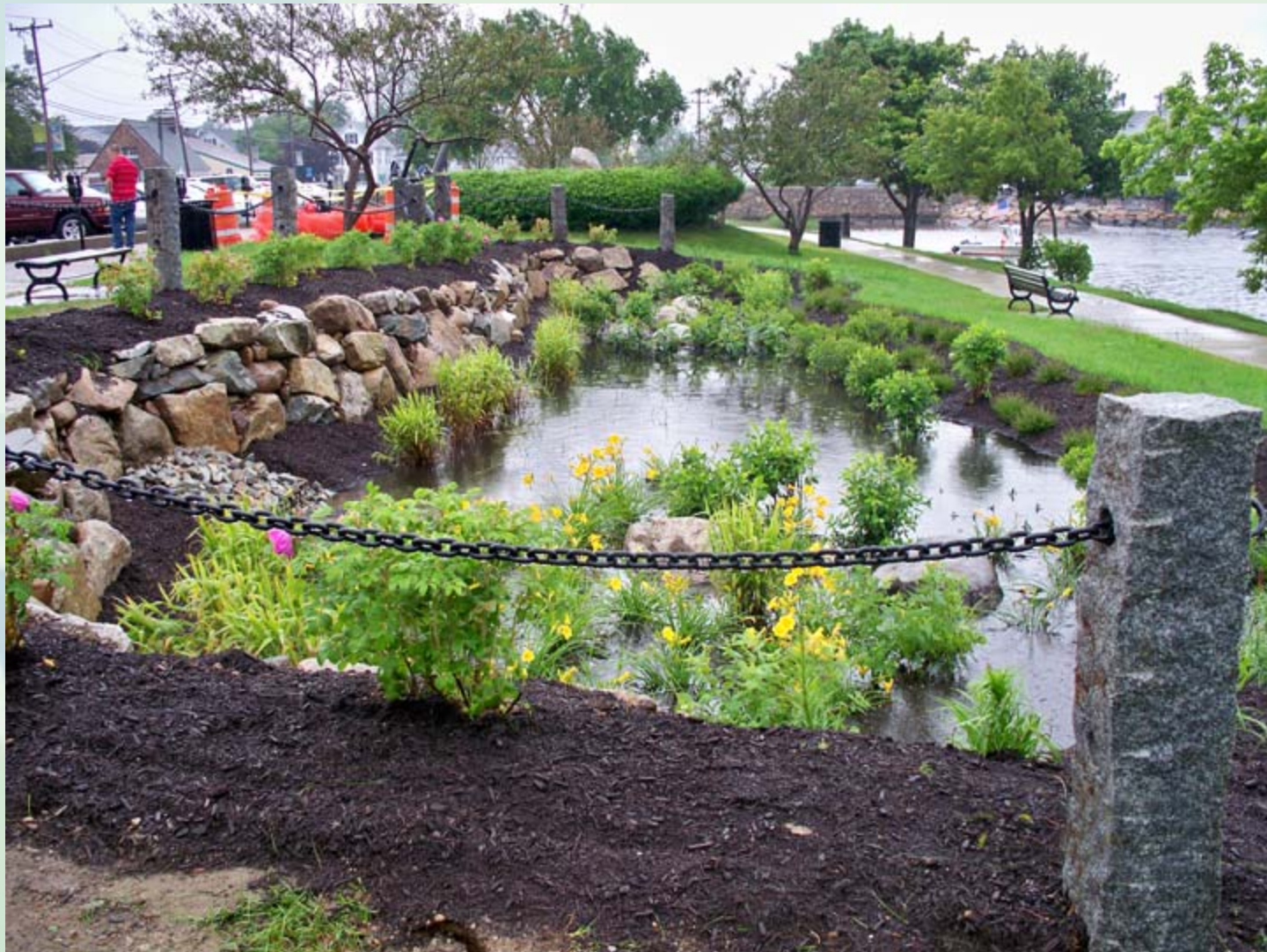
Bioretention Cell Water Street, Plymouth Center, MA
