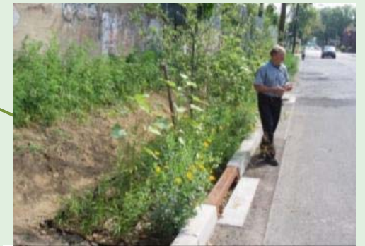
99 th Ave. street-side infiltration swale
