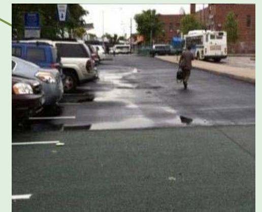
Far Rockaway porous pavement
