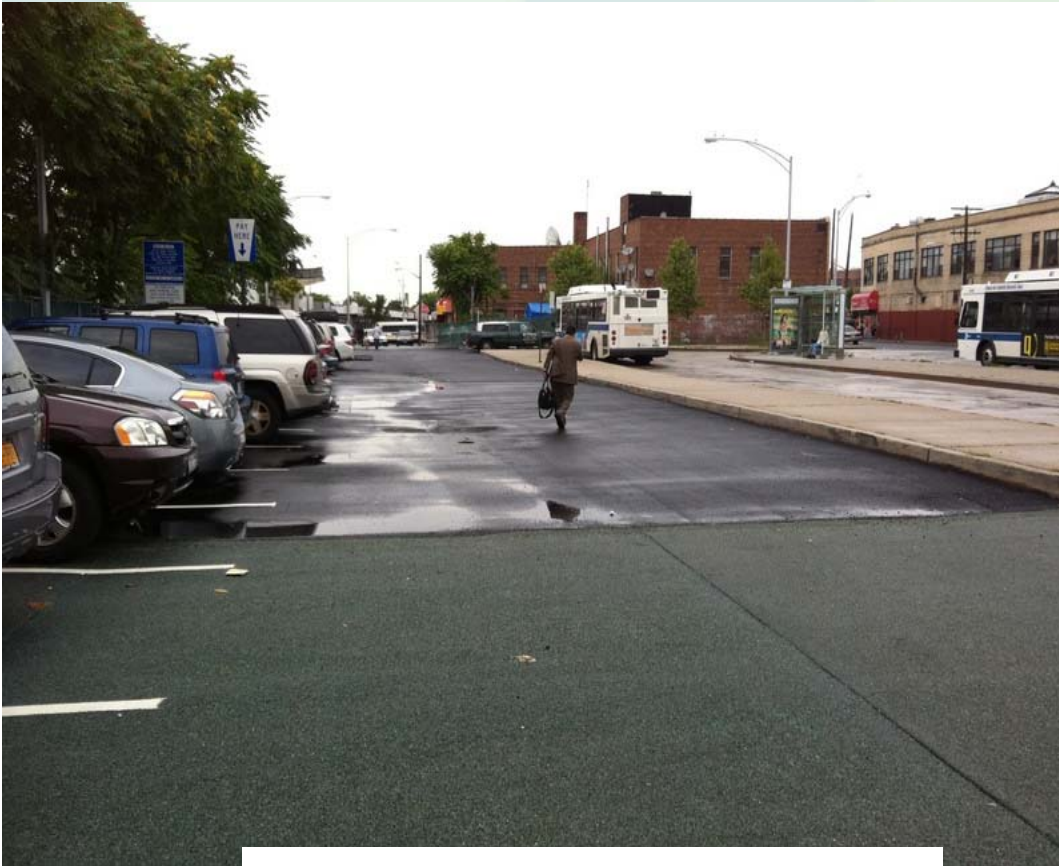
Permeable pavement
