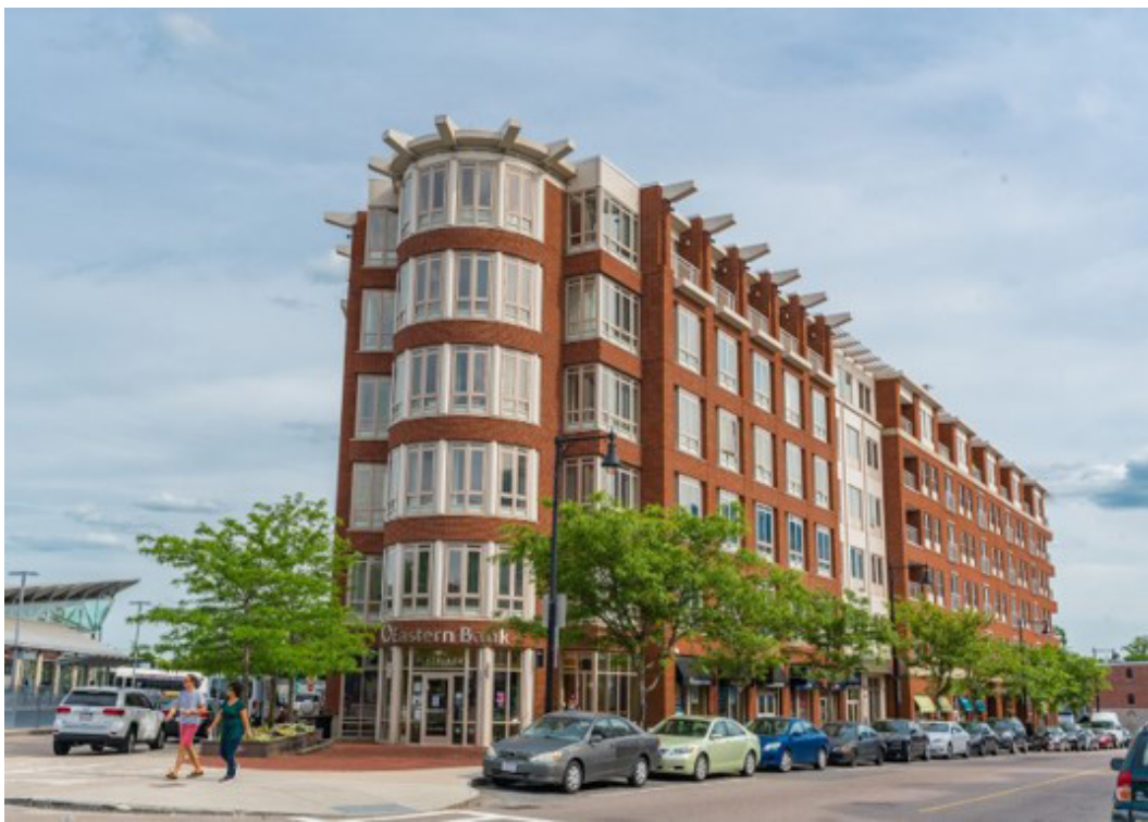
FIGURE 3: Past development on surplus MBTA property at Ashmont Station (c) Greater Ashmont Main Street
