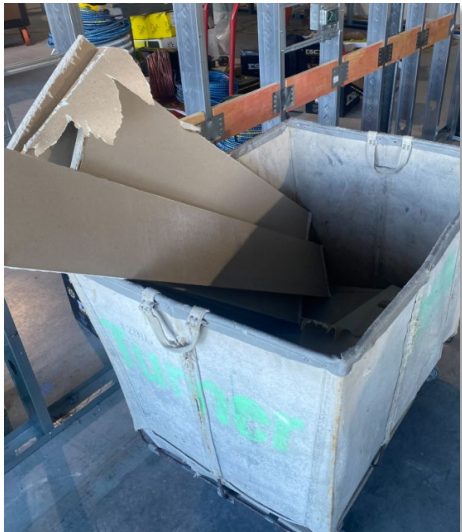
Clean GWB Offcuts
