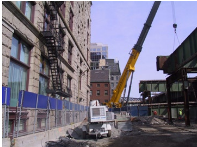
Looking north along Purchase Street facade of Grain Exchange
