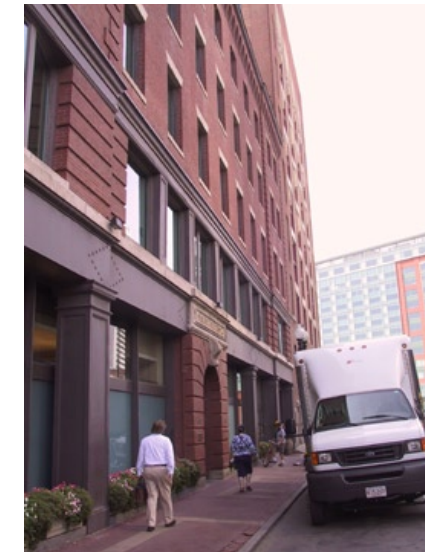
View of existing sidewalk looking south toward Independence Wharf
