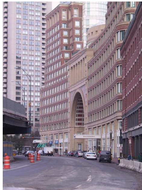
Existing condition at hotel entrance along Atlantic Avenue
