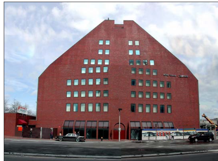
Marriott Long Wharf Hotel, Atlantic Avenue
