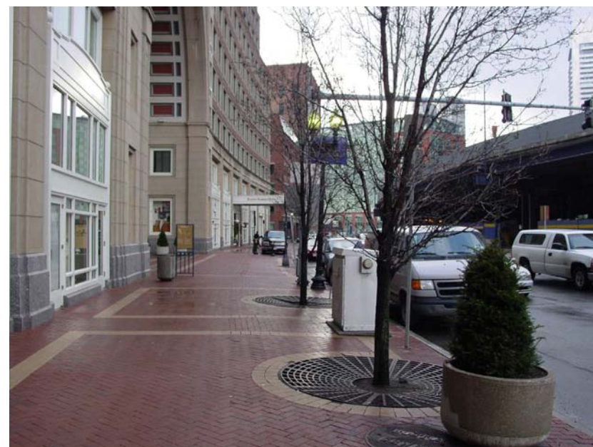
Existing sidewalk north of rotunda, +/- 20' wide
