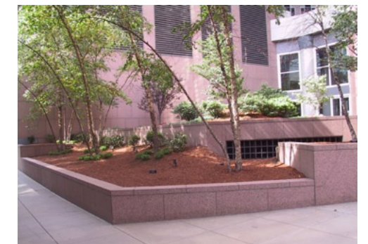
Existing elevated terrace and planter
