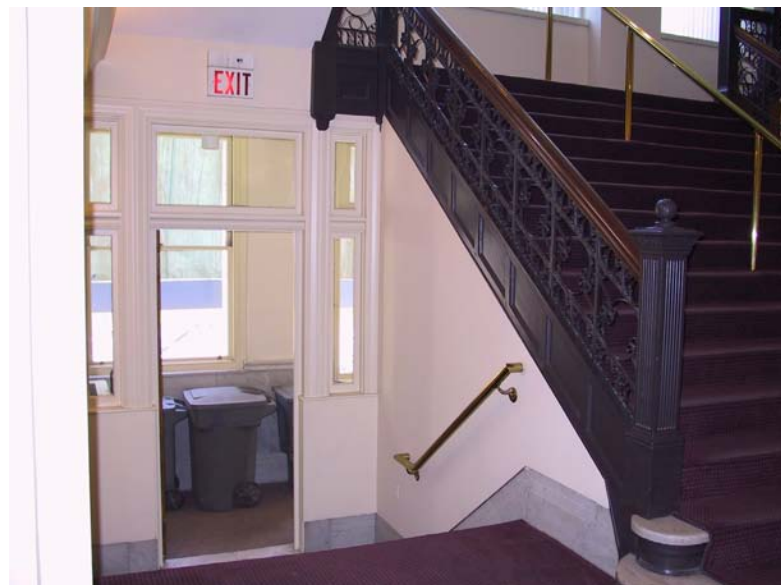
Main lobby level looking down to Purchase Street vestibule
