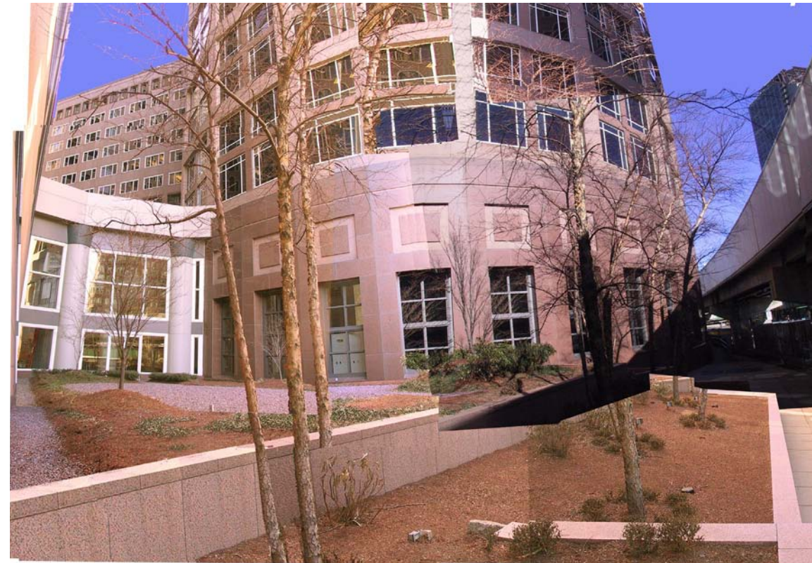
View of existing ballasted terrace between #1 and #2 International Place looking north up Purchase Street. The space offers potential for a new kitchen, entrance and outdoor seating area for a restaurant in Lobby #2.
