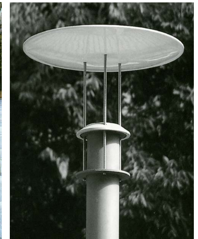
Pedestrian scaled lighting may be utilized to define the drop-off lanes and reduce the number of bollards required
