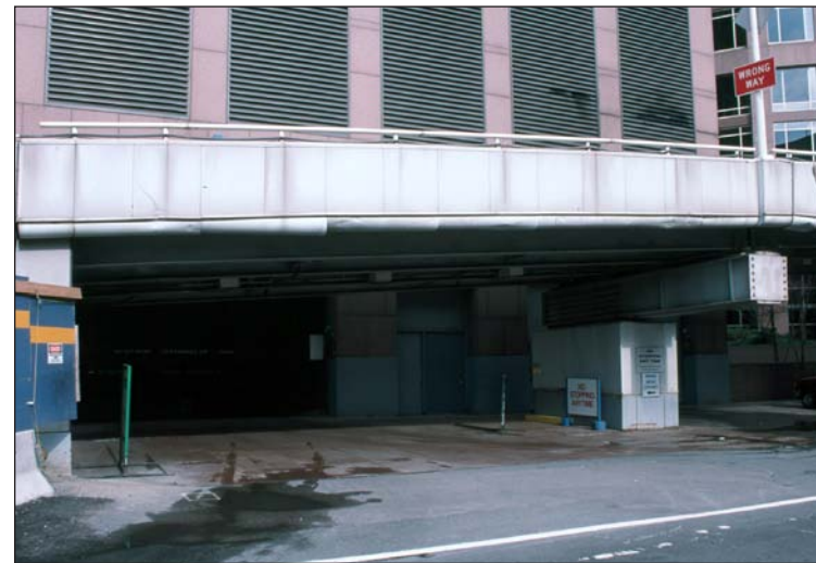
Parking entrance at Purchase Street
