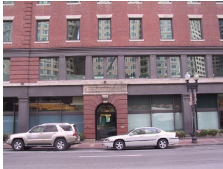
Façade of 400 Atlantic Avenue seen from the surface artery
