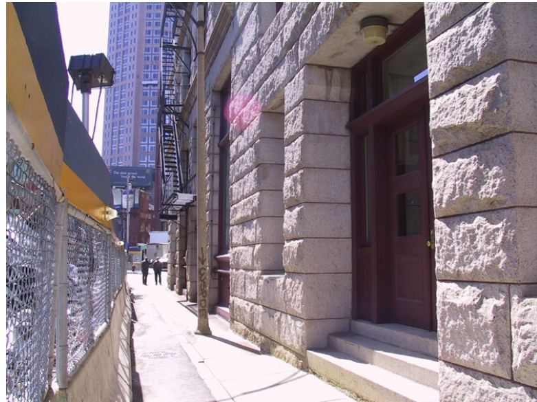
Existing rear entrance with steps up to vestibule level (El. +2'-4")
