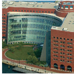
John Joseph Moakley Boston Federal Courthouse
