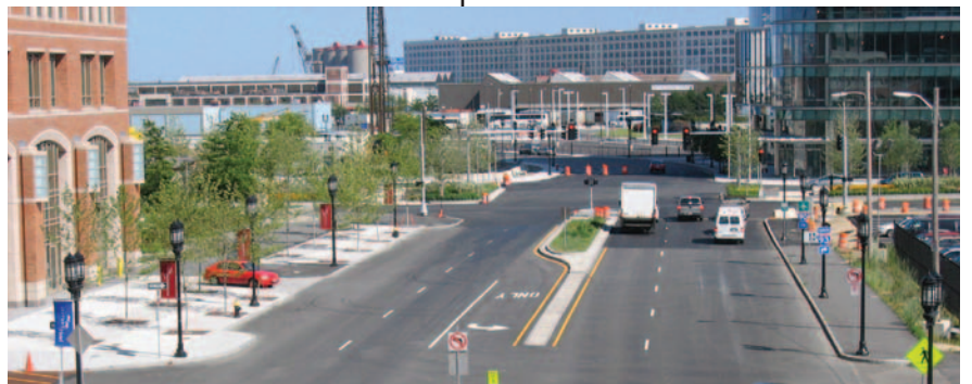
Within the Core Block area the streetscape is complete
