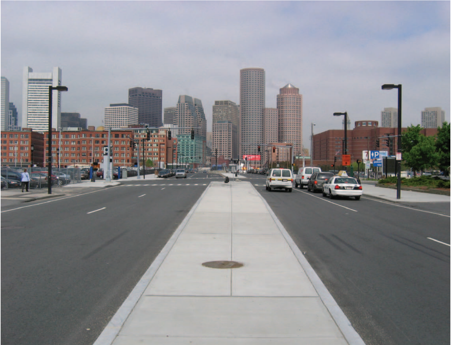
Existing view west along Seaport Boulevard
