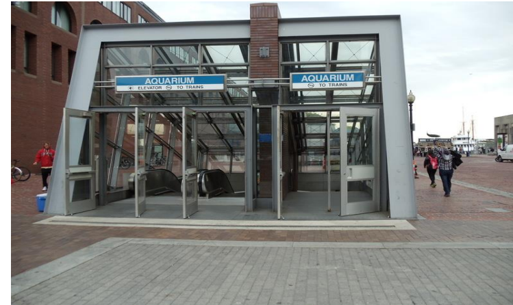
MBTA Aquarium Station-MBTAAQ
