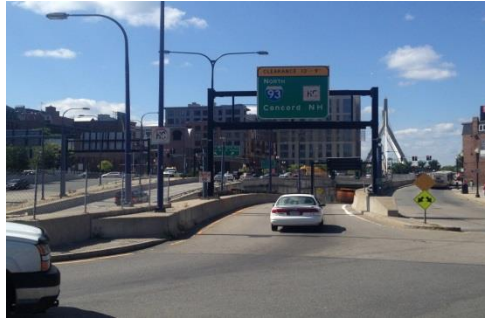
Tip O'Neill Tunnel Exit & Entrance Ramps
